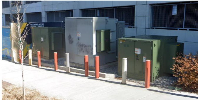
Radial Distribution Feeder Service
